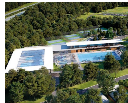
An artist impression of the $80 million Pimpama Sports Hub, scheduled for completion in 2020/21.
